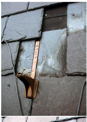
3) Attach the snow guard directly to the roof deck using nails or screws (copper or stainless steel).
