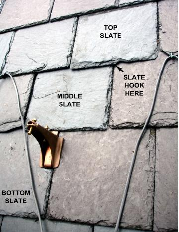
4) Slide the middle slate back into place after punching a second nail hole above the existing nail hole on the right side of the slate. Use these two nail holes to nail the slate into place. The top slate will need to be installed using a slate hook. Just nail the slate hook into place and slide the top slate back in and let it rest on the slate hook.
