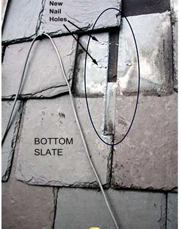
2) Notch the bottom slate on the top right side to allow room for the snow guard strap. Before notching, punch two new nail holes as shown, using either a slate hammer punch, or a punch on a slate cutter. After notching the slate with the slate cutter, nail it back in place using two nails on one side.
